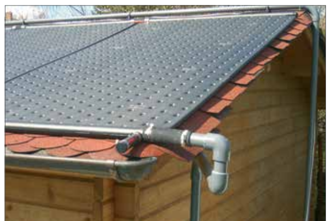
Sloping roof installation
