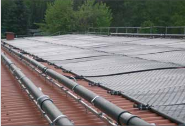
Flat roof installation
